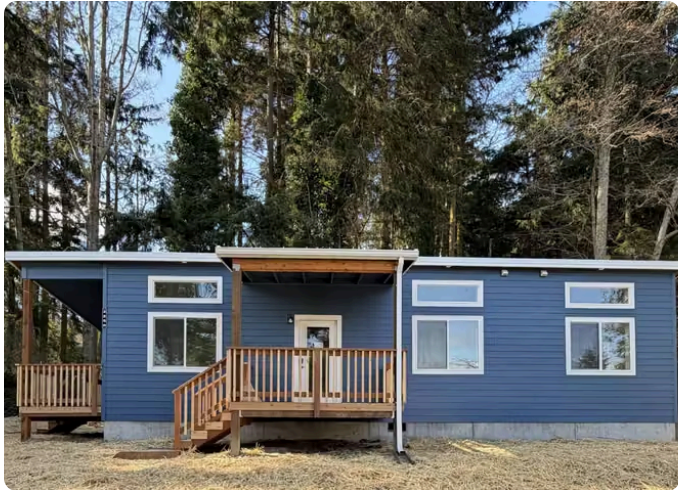
A completed Model F; selections and site improvements vary.
