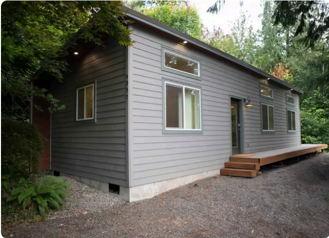
A completed Model E; selections and site improvements vary.
