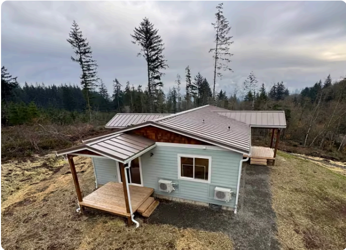
A completed Model I; selections and site improvements vary.
