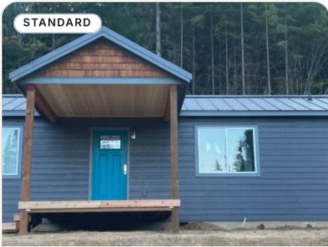
Lap siding Fiber-cement lap siding, painted in the colors you choose.
