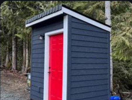
Well pump house
