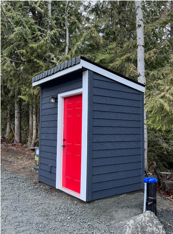
WELL PUMP HOUSE
