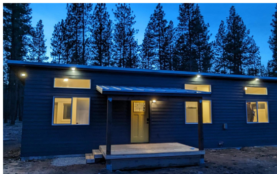
EXTERIOR SOFFIT LIGHTS Upgrade - Minimum of 3 required
