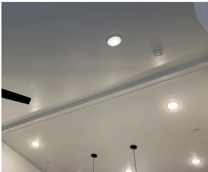
DRYWALL WRAPPED Upgrade
