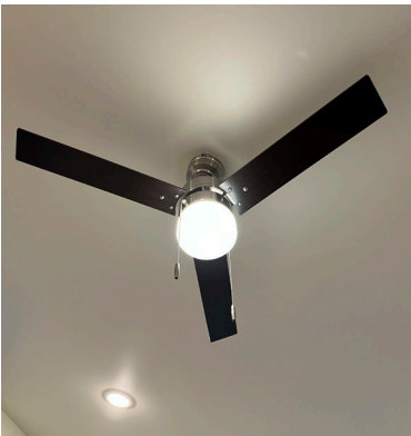
CEILING FINISH - SHEETROCK
