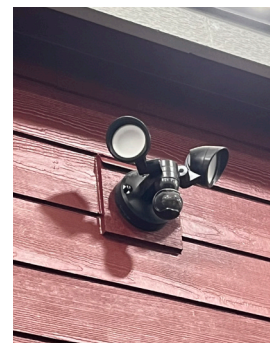
FLOOD LIGHT Upgrade
